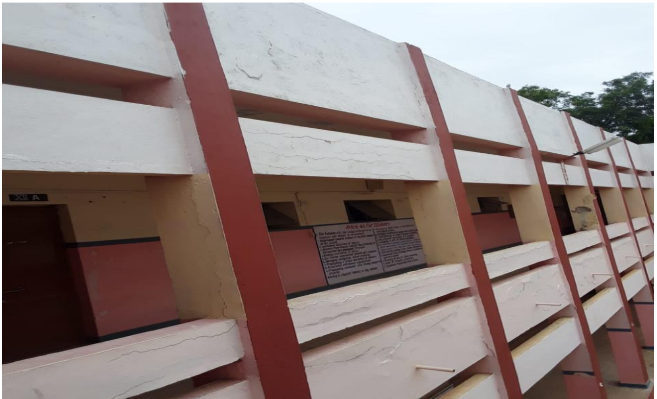
Figure 16: Major damages in the RCC member of School building
