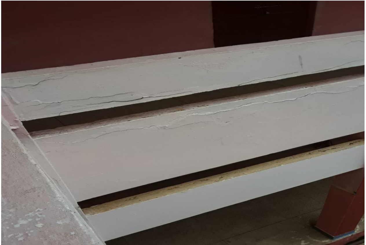
Figure 14: Damage in the inside passage area of old school building beam
