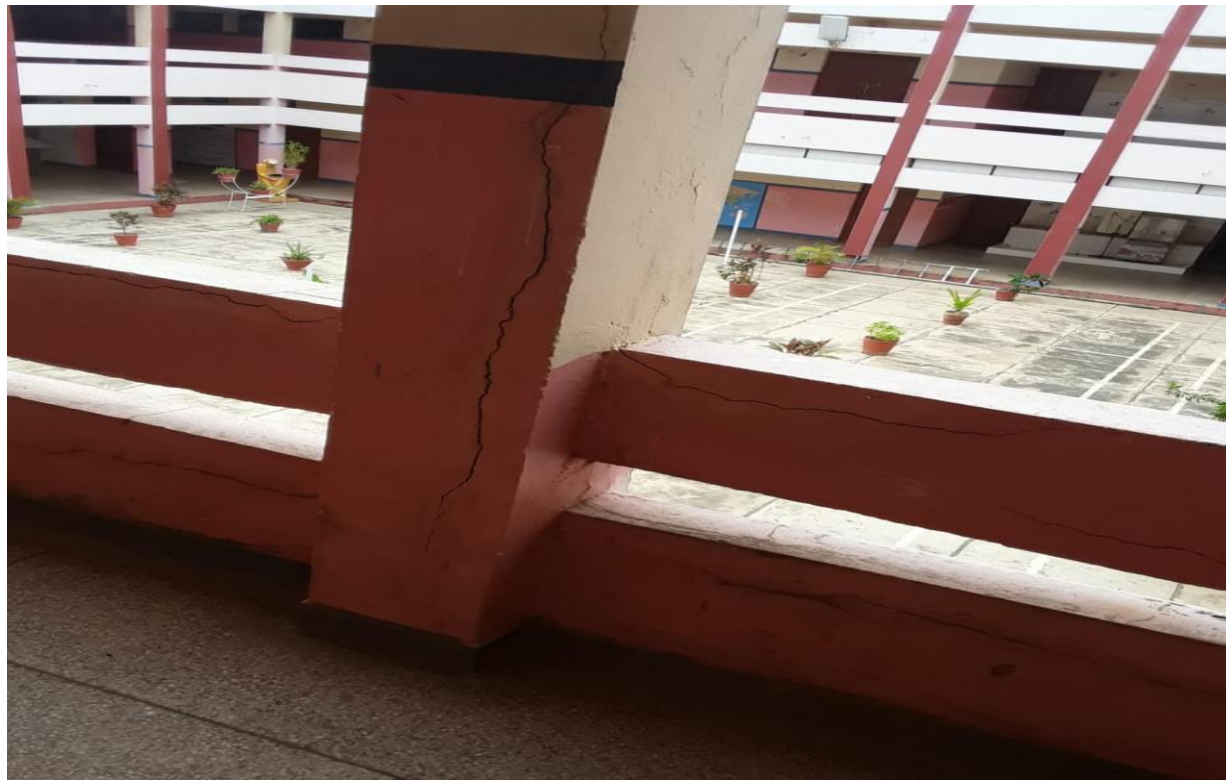
Figure 12: Structural Damage in the Column of old school building
