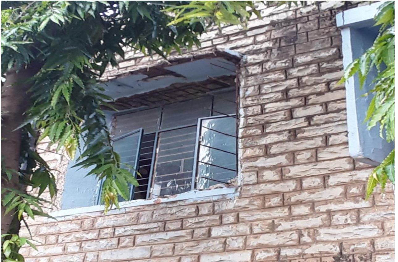
Figure 18: Reinforced bars exposed to open environment in a backside school building
