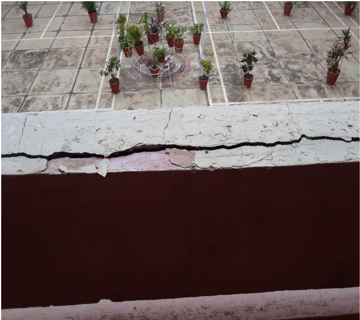
Figure 11: Structural Damage in the beam of old school building
