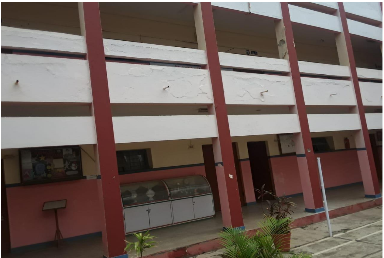
Figure 15: Structural Damage in passage area of old school building (Block A)
