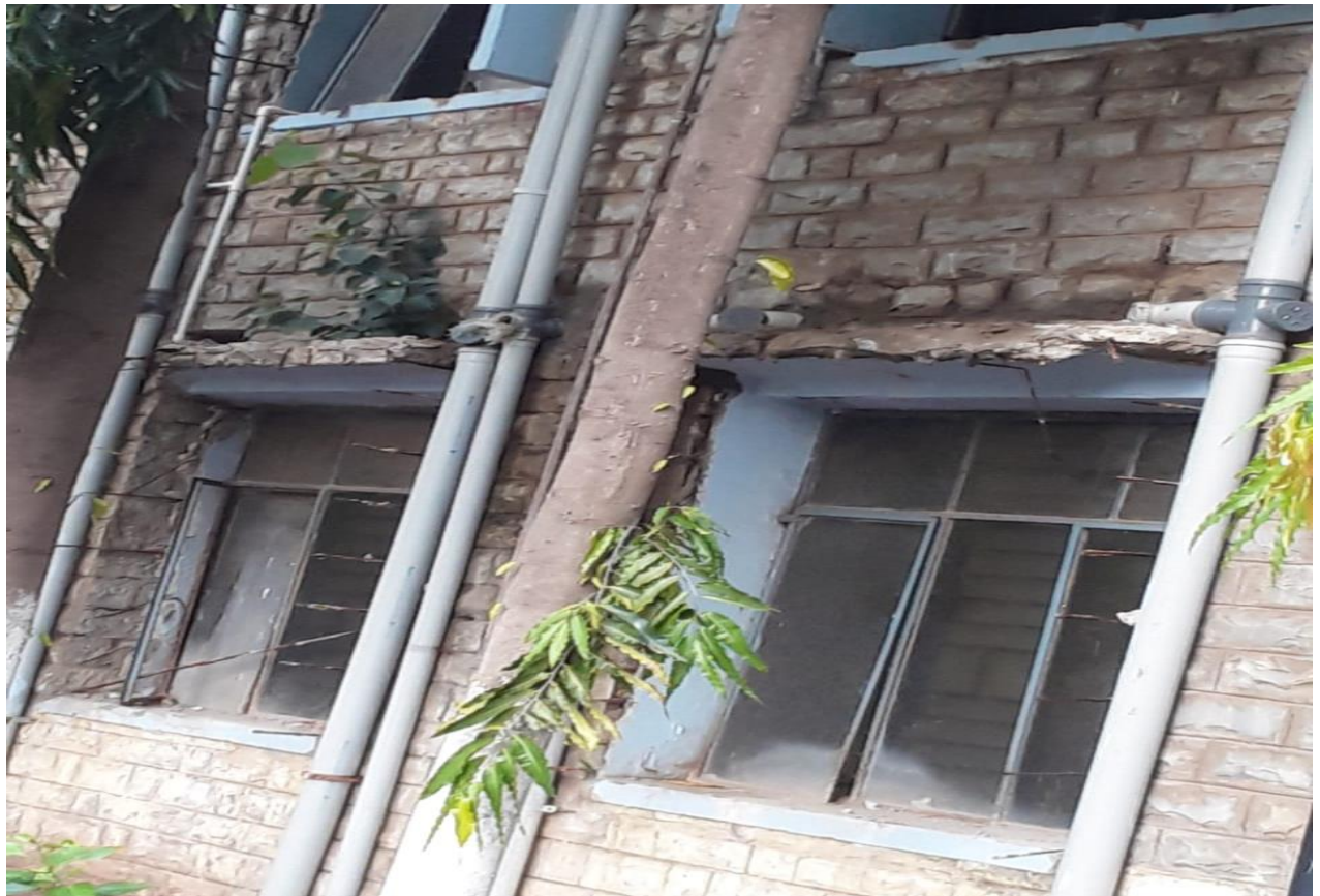
Figure 19: Damages in the projection of windows backside school building
